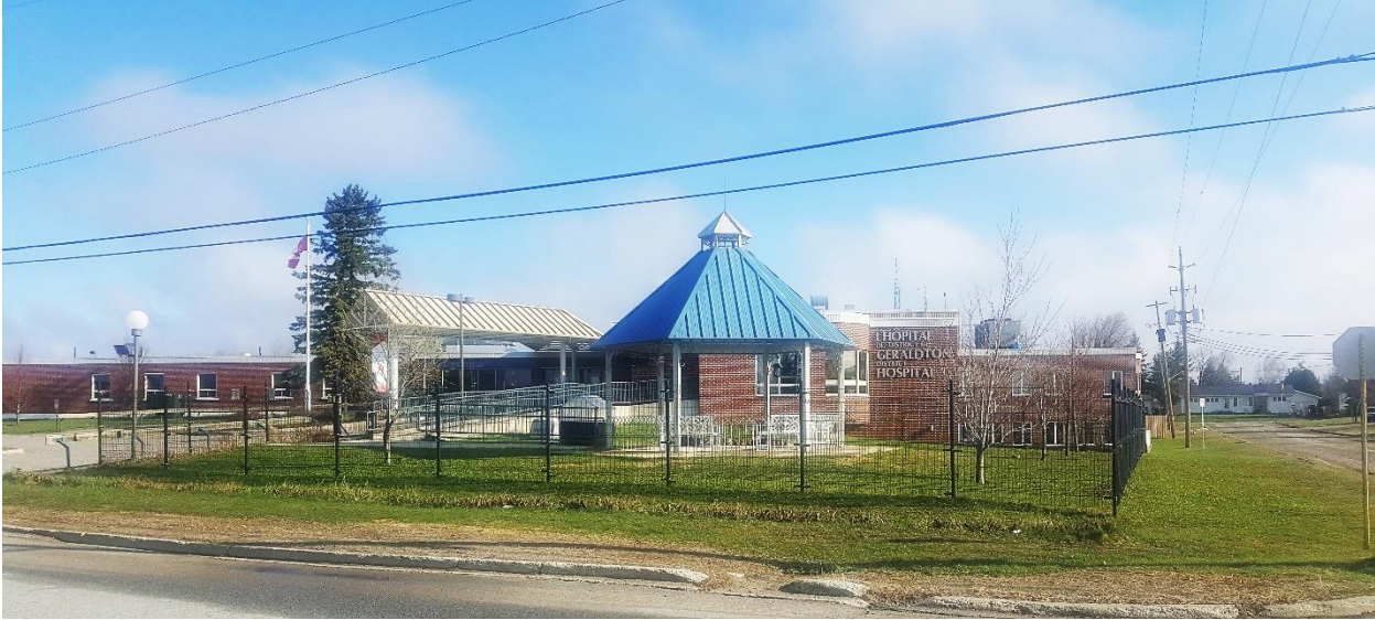
Picture 1. Geraldton District Hospital
