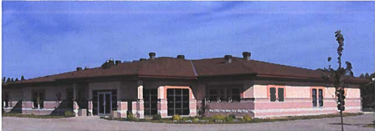
Picture 1. Geraldton District Hospital
