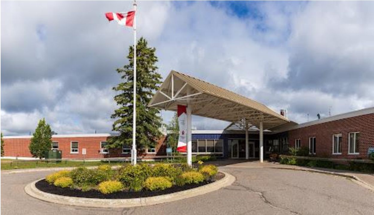
Figure 2. Geraldton District Hospital
